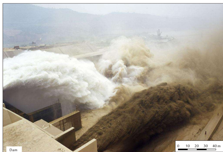
Fig. 1 Gates near both the top and the bottom of the reservoir dam of the Xiaoliandi Reservoir Lake were opened when a disastrous flood of the Yellow River threatened to overflow the dam. Huge water masses could thus be released. The water released from the top part of the lake, flowing through the upper gates of the dam, was clean. Due to mixing with air, this water was bright white. In contrast, the water released through the gates near the bottom had a brown color. This water was sediment-laden because a long-lived hyperpycnal flow eroded and whirled up much sediment from the reservoir's bottom. (From Yang et al. 2018, after https://www.quanjing.com/imgbuy/QJ8103941831.html )
