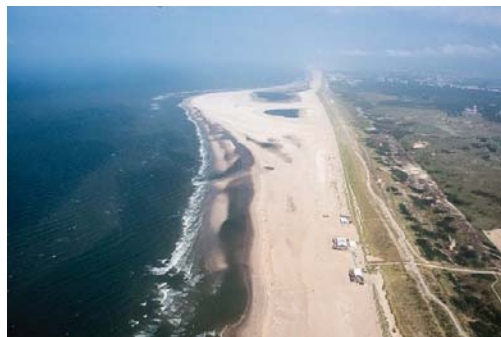
Figure 1. Aerial picture of the Sand Engine in September 2014, looking in northeasterly direction. This km-scale nourishment, with 21.5 \text{ Mm}^3 larger than regular nourishments ( 1\text{-}2 \text{ Mm}^3 ), was constructed in July 2011 along the southwest-northeast oriented Delfland coast, The Netherlands, as a sustainable and nature-based protection measure against coastal erosion (Stive et al., 2013). Courtesy: Rijkswaterstaat, Joop van der Hout.
