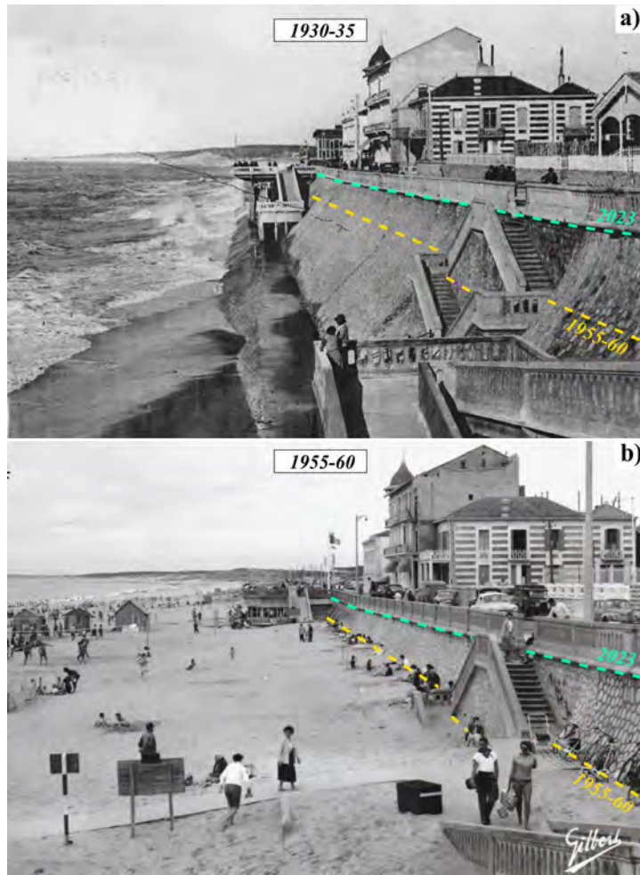
Figure 2: Historical photographs of Soulac-sur-Mer seafront a) in the early 1930s and b) late 1950s, showing the dramatic elevation and widening of the beach. In the 1930s, the beach level was at the foot of the sea wall. This sandy beach rose several meters to reach the yellow dotted line in the late 50s. In 2023, the beach level is at the cyan dotted line.
