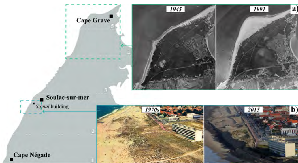
Figure 3: Historical aerial photographs illustrating the large-scale shoreline evolution, accreting sector in the north (1945-1991) and eroding sector south of Soulac-sur-Mer, in front of the Signal building (1970s-2015). (Ph. 1970s, source unknown; Ph. 2015, @L.Theillet)
