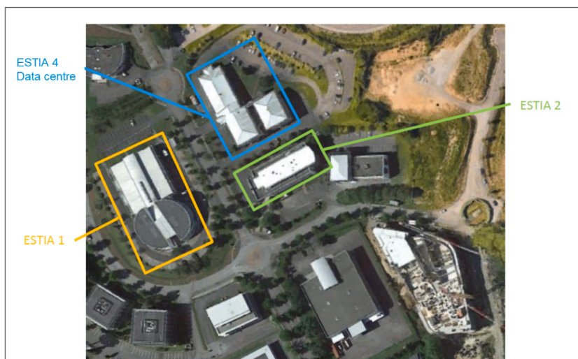
Fig. 1. The three buildings involved in the CSC of Izarbel technology park.
