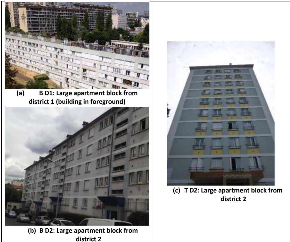
Figure 4 : Picture of the three studied representative buildings. Photo credits: OPHM.
