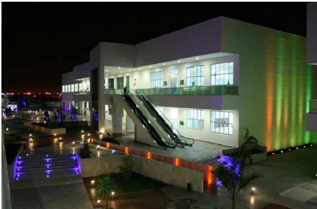
Figure 2. Building of Business Incubator. Cultural Complex of the Autonomous University of Puebla
